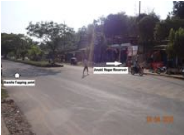
Typical transmission pipeline route
