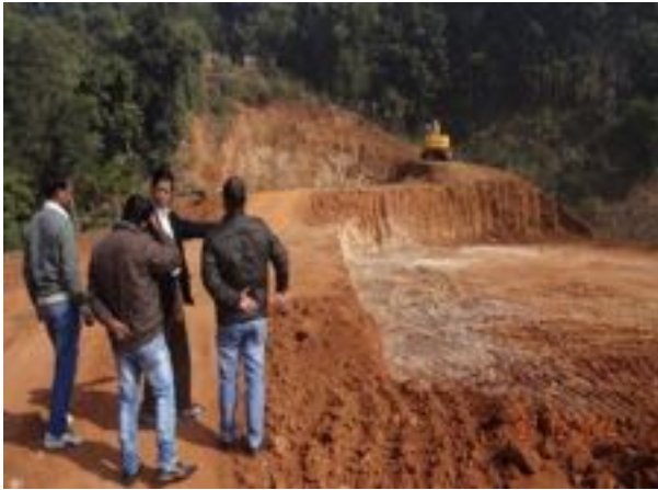
Gopal nagar reservoir site- reservoir under construction
