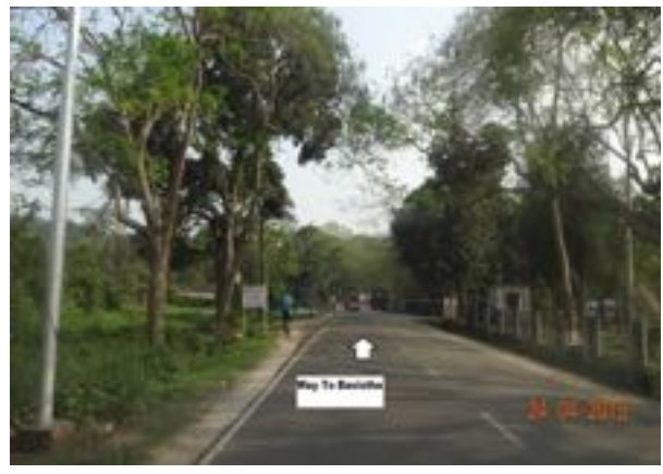
Typical transmission pipeline route
