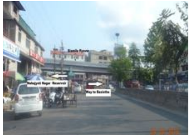
Typical transmission pipeline route
