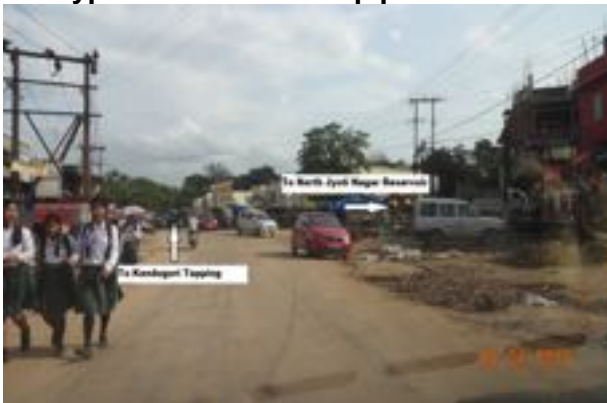
Typical transmission pipeline route
