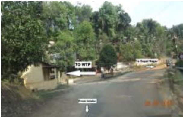
Typical transmission pipeline route
