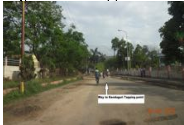
Typical transmission pipeline route
