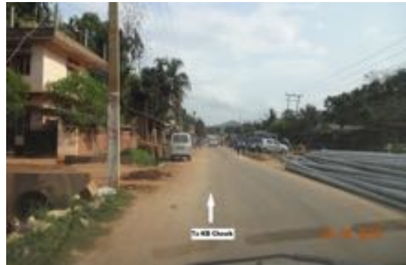
Typical transmission pipeline route
